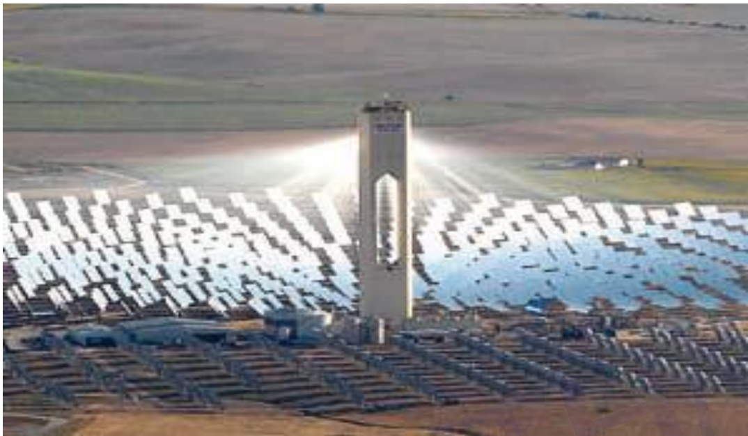
Figure 2.10: Heliostat field collectors (Marc et al., 2010)
