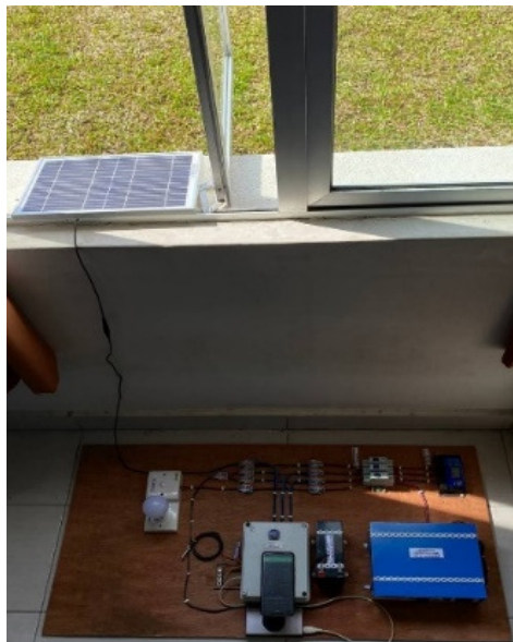
FIGURE 10. Outdoor solar system testing
