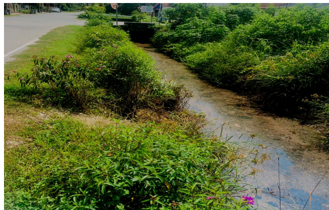
Figure 2. Current condition of the drainage system
