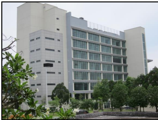
Figure 1.1: NIOSH Tower building in Bandar Baru Bangi, Selangor
