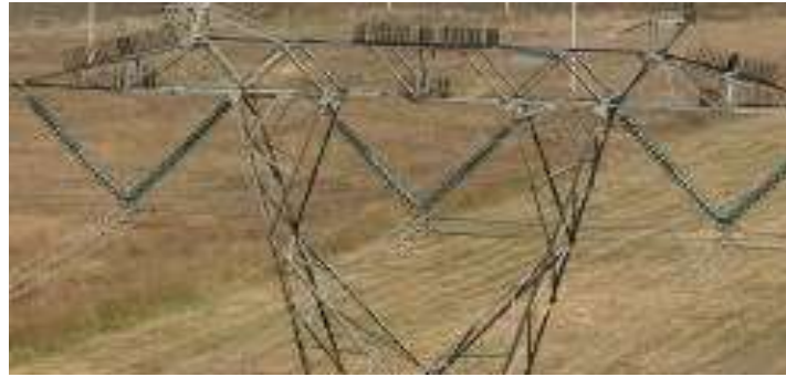
Figure 2.2: V-V-V assembly on 433B tower after re-insulation [8].
