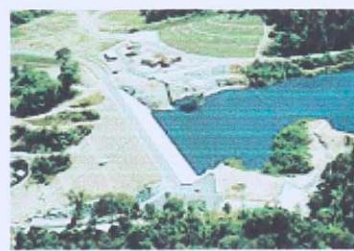
Beris Dam, Kedah (completed in 2003)
