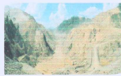
Bakun Dam, Sarawak (expected to complete in 2009)
