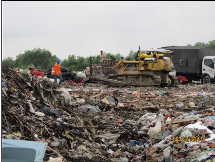
Figure 6: Levelling activity using bulldozer
