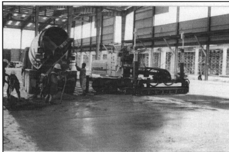
Figure 5 Construction SFRC slab in Giant Hypermarket
