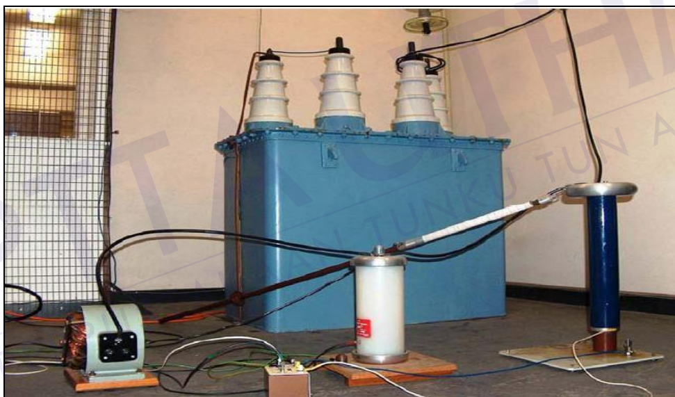
Figure 1.3 On lab - partial discharge measurement
