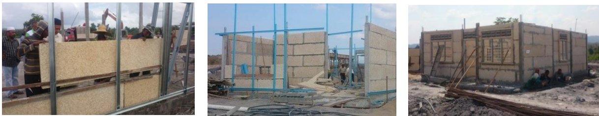
Figure 1. Current construction practiced using WWCP as wall element (Duralite (M) Sdn. Bhd.)
