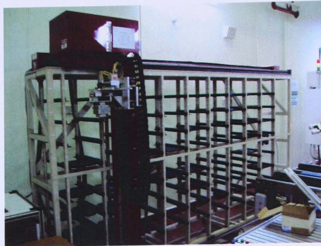
Figure 3.4: The Racking and SRM
