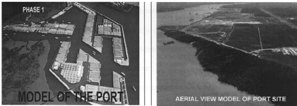
FIGURE 4 : Views of model of Port Tanjung Pelepas site (Courtesy of IEM Magazine, 1999)
