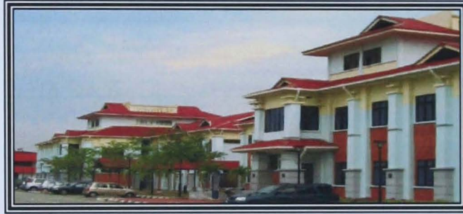
Figure 1.2: Front view of Lecturer Block C15 and C16.
