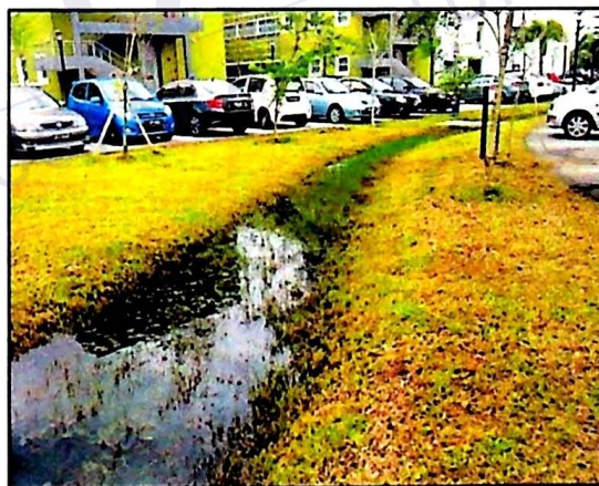
Figure 1.1 : Grassed swale adjacent to parking lot in UTHM
