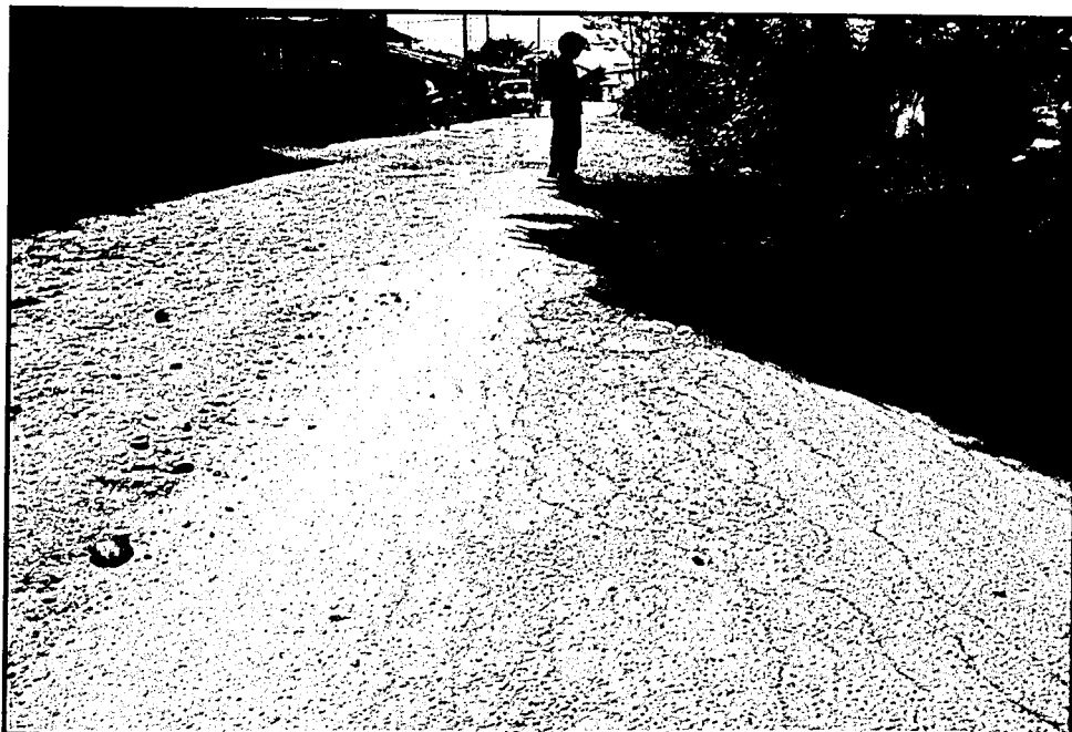
Figure 2.5: Typical Fatigue Cracking on Road Pavement Surface (Jestin, 2006)
